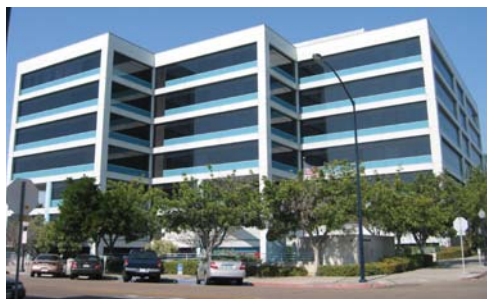
The presence of the Police Department headquarters (above) and Fire Department station benefit public safety efforts, but additional police and fire stations will be needed to maintain service levels in future years.
