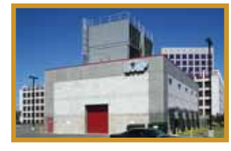
27 Harbor Drive Pedestrian Bridge Pedestrian Bridge
