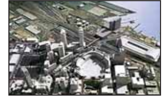
26 East Village District Plant Central Cooling Plant
